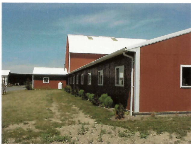
Gutters on farm buildings divert clean water away from barnyard areas, reducing the removal of barnyard wastes.
