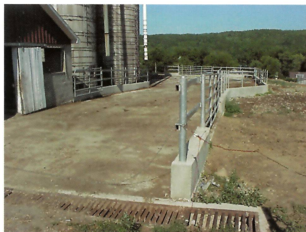
Concrete barnyards allow easy removal of manure and other barnyard wastes and make it easier to control runoff.
