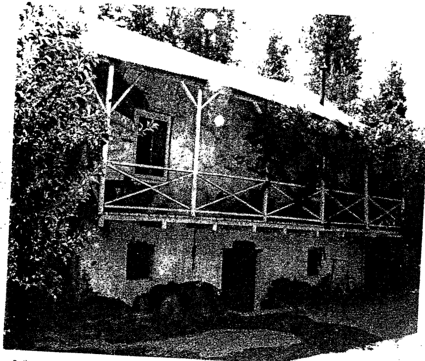
Built in 1872, the old Fossati winery now serves as the tasting room for the Boeger Winery, just east of Placerville in the picturesque Apple Hill district. The historic
